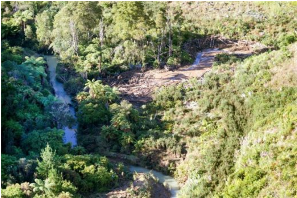
Slip adjacent to tributary into Cosseys Reservoir
