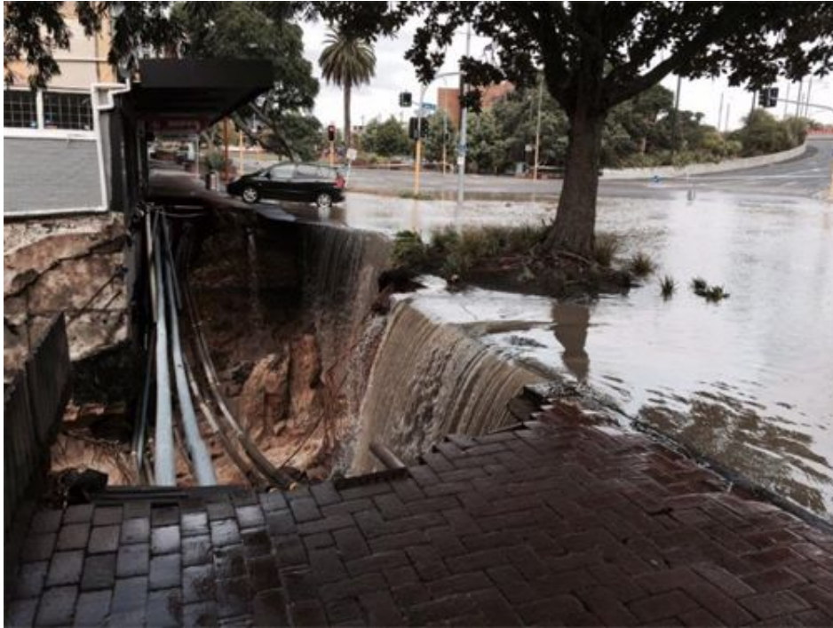
Sinkhole at Great North Rd, New Lynn
